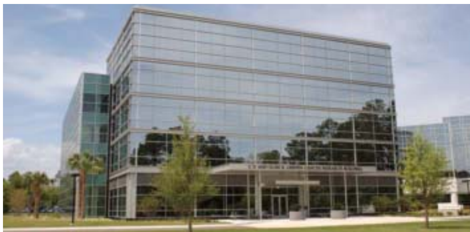
Pictured is the new C.V. and Elsie R. Griffin Cancer Research Building at Mayo Clinic in Jacksonville. The building was dedicated in February. The center is named after C.V. and Elsie R. Griffin, longtime Mayo Clinic patients and benefactors, whose gift along with a host of others contributed to the construction of the $22 million building.
